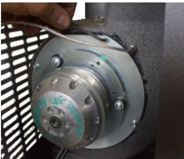
Fig. 42 - Exhaust fan cleaning: stage 1
