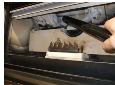
Fig. 38 - Upper part cleaning
