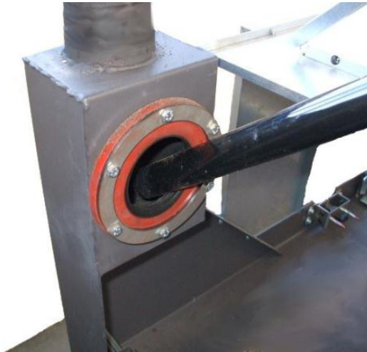
Fig. 41 - Fume pipe cleaning
