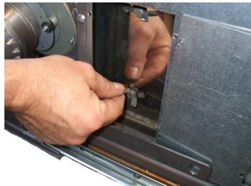
Fig. 46 - 2° panel removal
