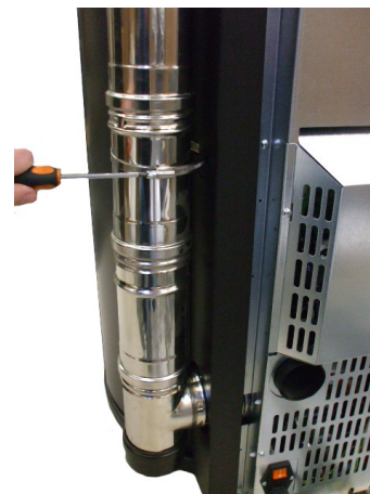
Fig. 75 - Rookleiding (Sfera 3 Plus, Sfera 3 , Globe, Elise 3 Plus)
