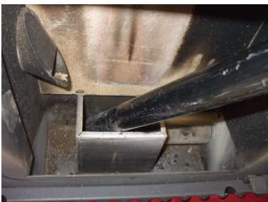
Fig. 30 - Burning pot box cleaning
