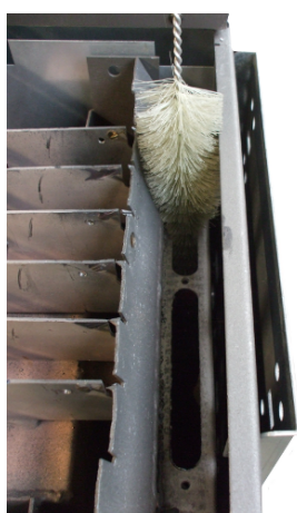
Fig. 43 - Fume passages cleaning
