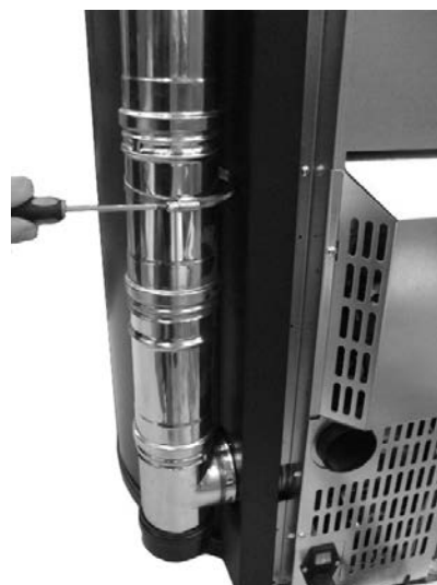
Fig. 103 - Rookleiding (Sfera 3 Plus, Sfera 3 , Globe, Elise 3 Plus)
