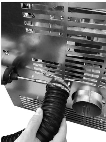
Fig. 12 - Raccordement air comburant
