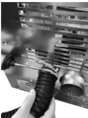
*Fig. 11 - Raccordement air comburant*
