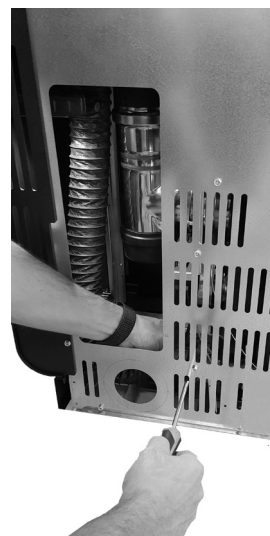
Fig. 57 - Raccorder le tuyau flexible
